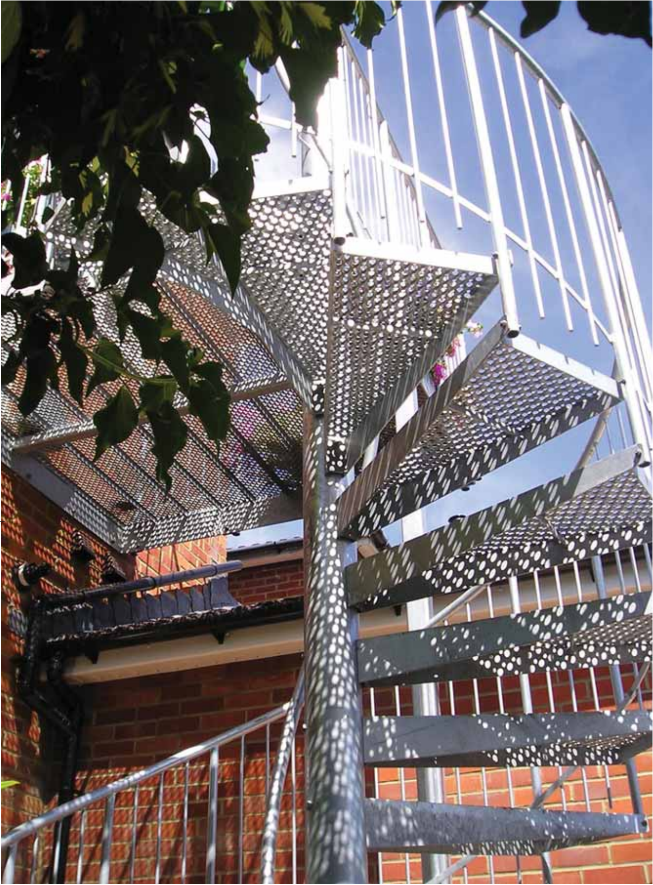
Main picture: Domestic fire escape and balcony with non slip perforated treads and deck.
