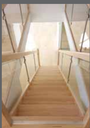
Bottom right: Half turn traditional stair in maple. Large mid platform and glass panels.
