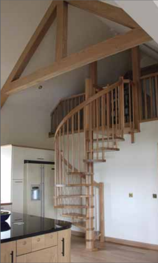
Top right: Model 77 spiral Staircase with oak treads. Centre column 5 x stainless cylinders.
