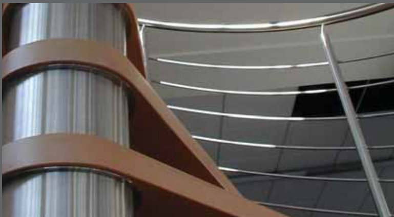
Bottom left: Model 73 spiral Staircase. Detail showing the brushed stainless steel centre column.
