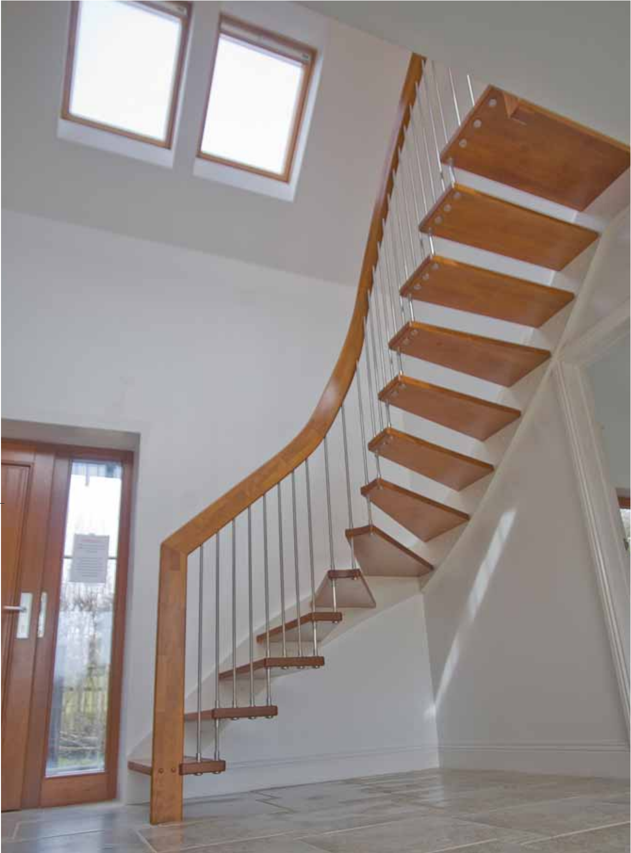
Main picture: Quarter turn WF Staircase with beech treads. White wall stringer and curved internal handrail.
