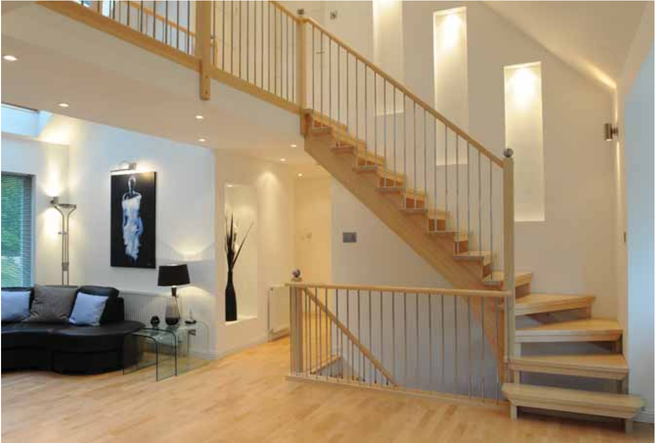
Main picture top: Quarter turn maple stepped style Staircase with stainless steel spindles.
