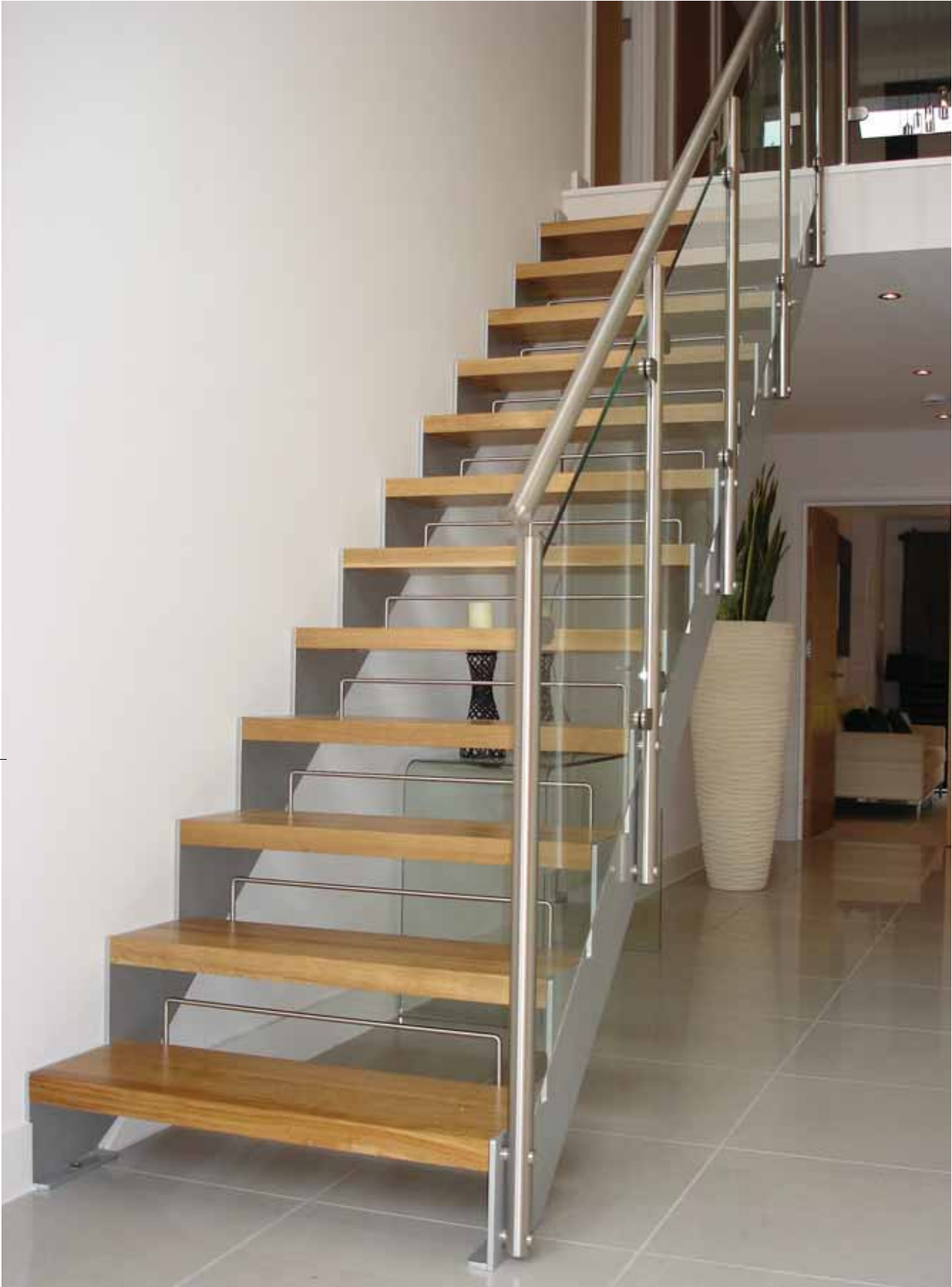
Main picture: Straight flight Model 500 Staircase with oak treads, glass balustrade and stainless riser bars.
