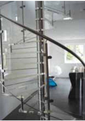
Bottom right: Model 76 with acrylic treads and curved acrylic balustrade panels.
