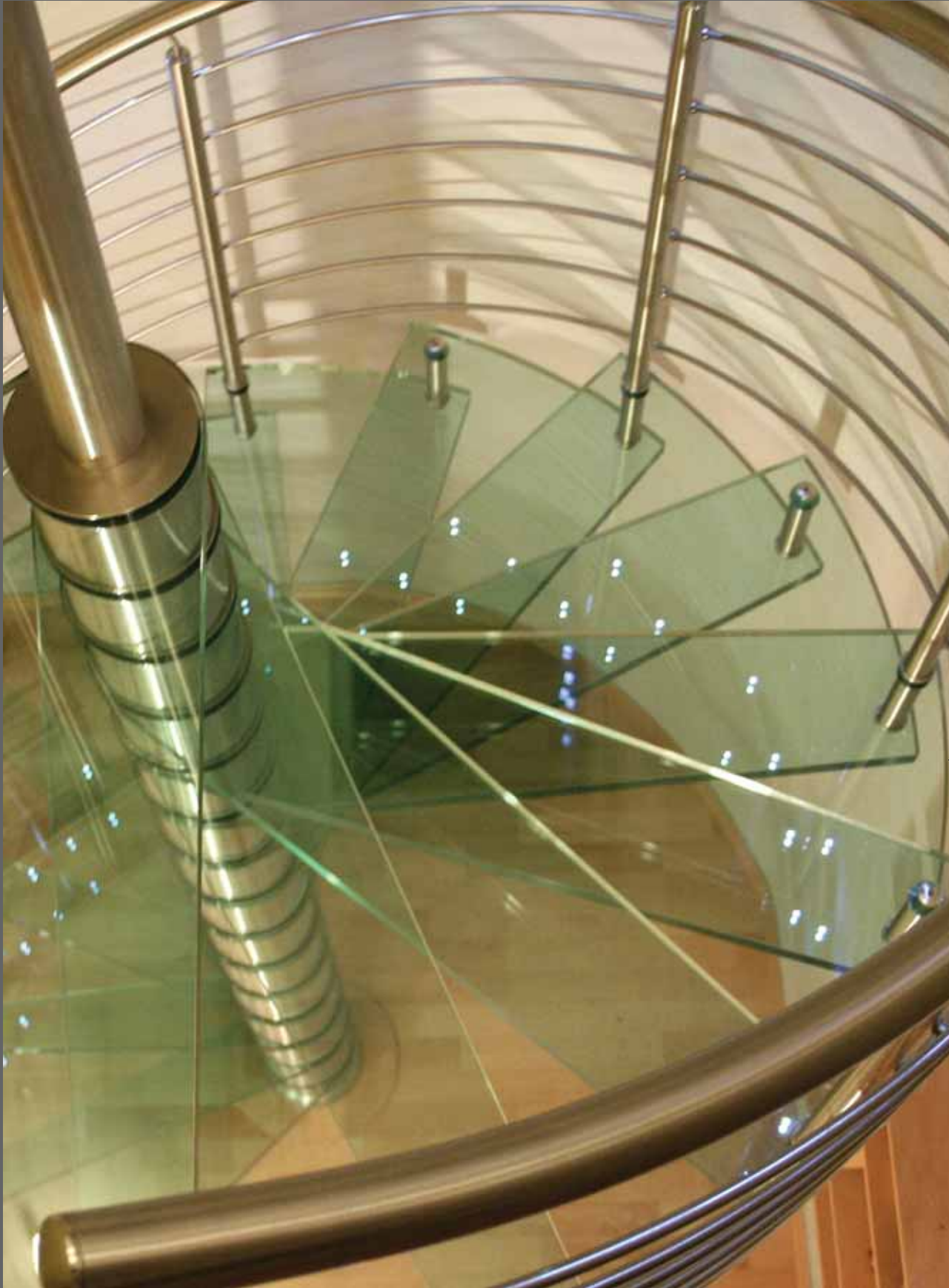
Bottom left: Detail of the brushed stainless steel centre column on the Model 76.
