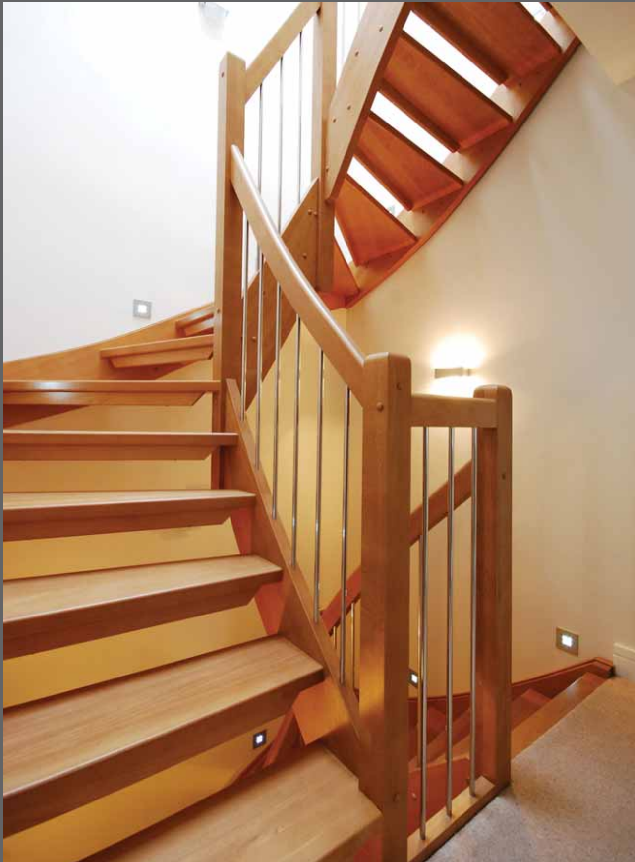
Main picture: Half turn traditional stair in beech with stainless spindles and open risers.
